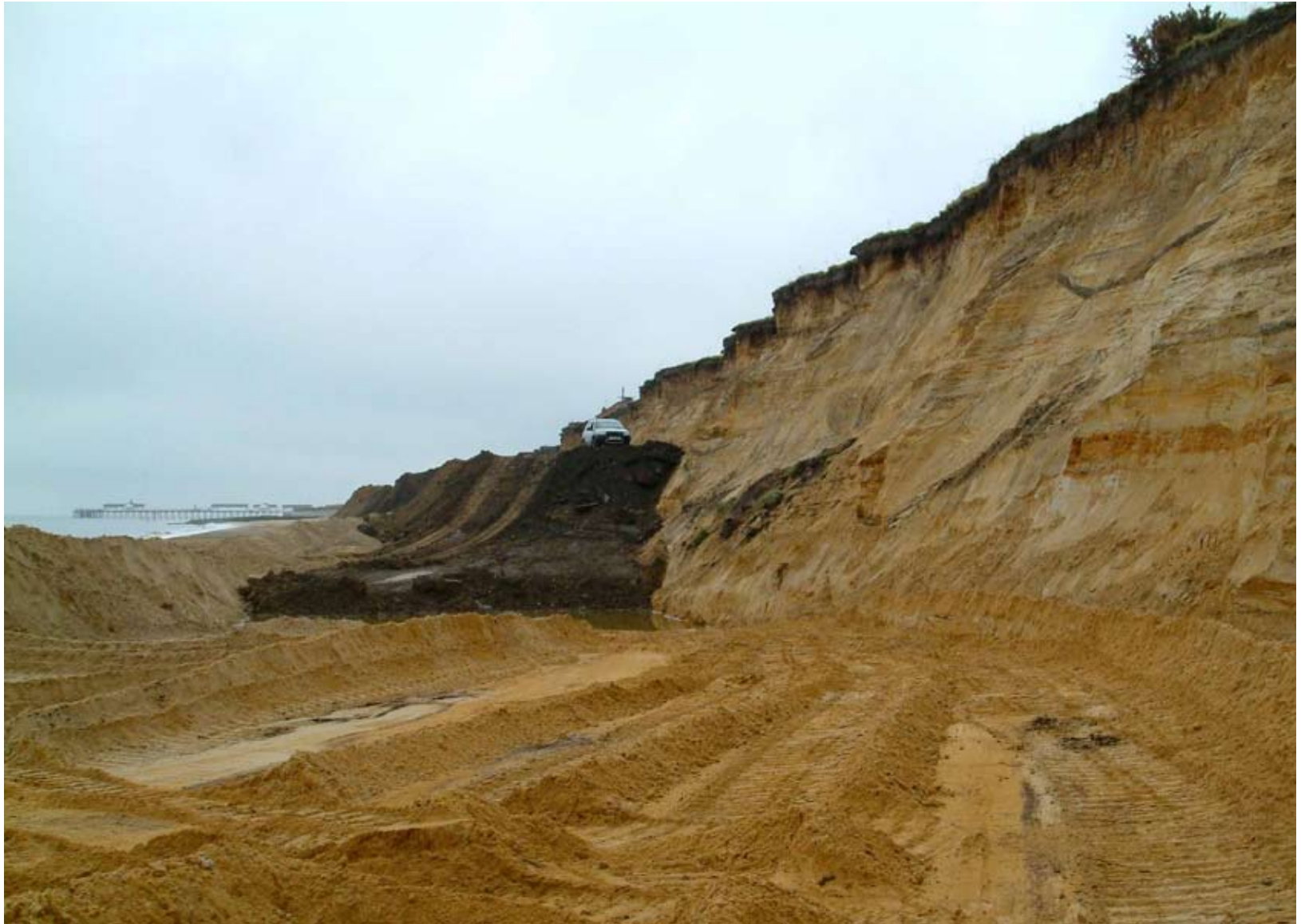
Simon Read, Reclamation works at Easton Bawents , 2005.
