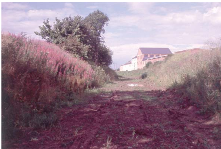
Dry Canal Bed & Industrial Buildings, Cropwell Bishop
